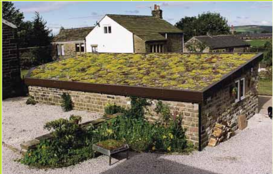
100sqm Nature Roof fully installed in a day (11 months old)
