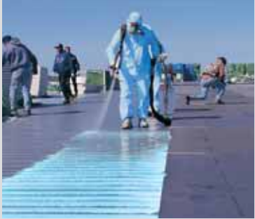
Flexible FAST Adhesive is applied to metal deck
