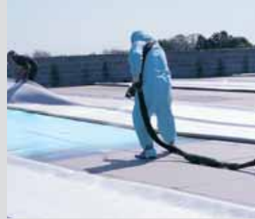
Flexible FAST is spray applied to insulation
