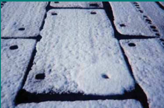
Flexible FAST can eliminate thermal bridging of the fasteners and insulation joints that is causing the snow to melt and draining energy from the building.
