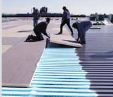
Insulation is set into Flexible FAST Adhesive
