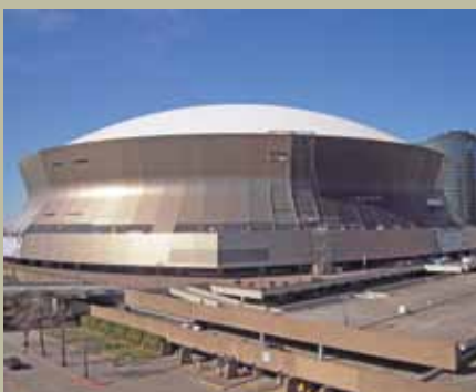
Louisiana Superdome, New Orleans, USA
