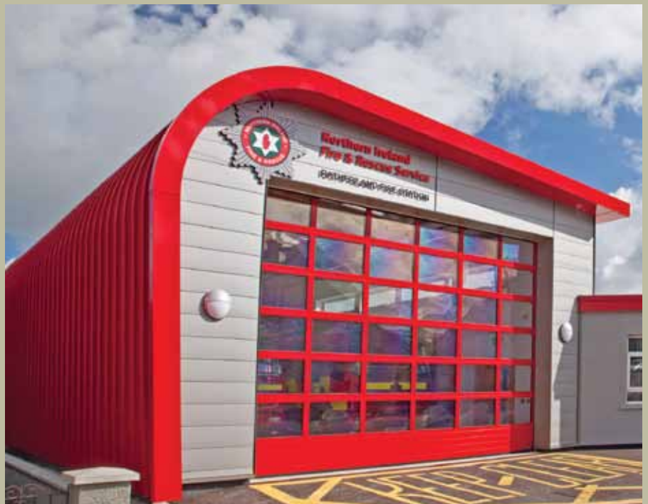
Rathfriland Fire Station, Northern Ireland
